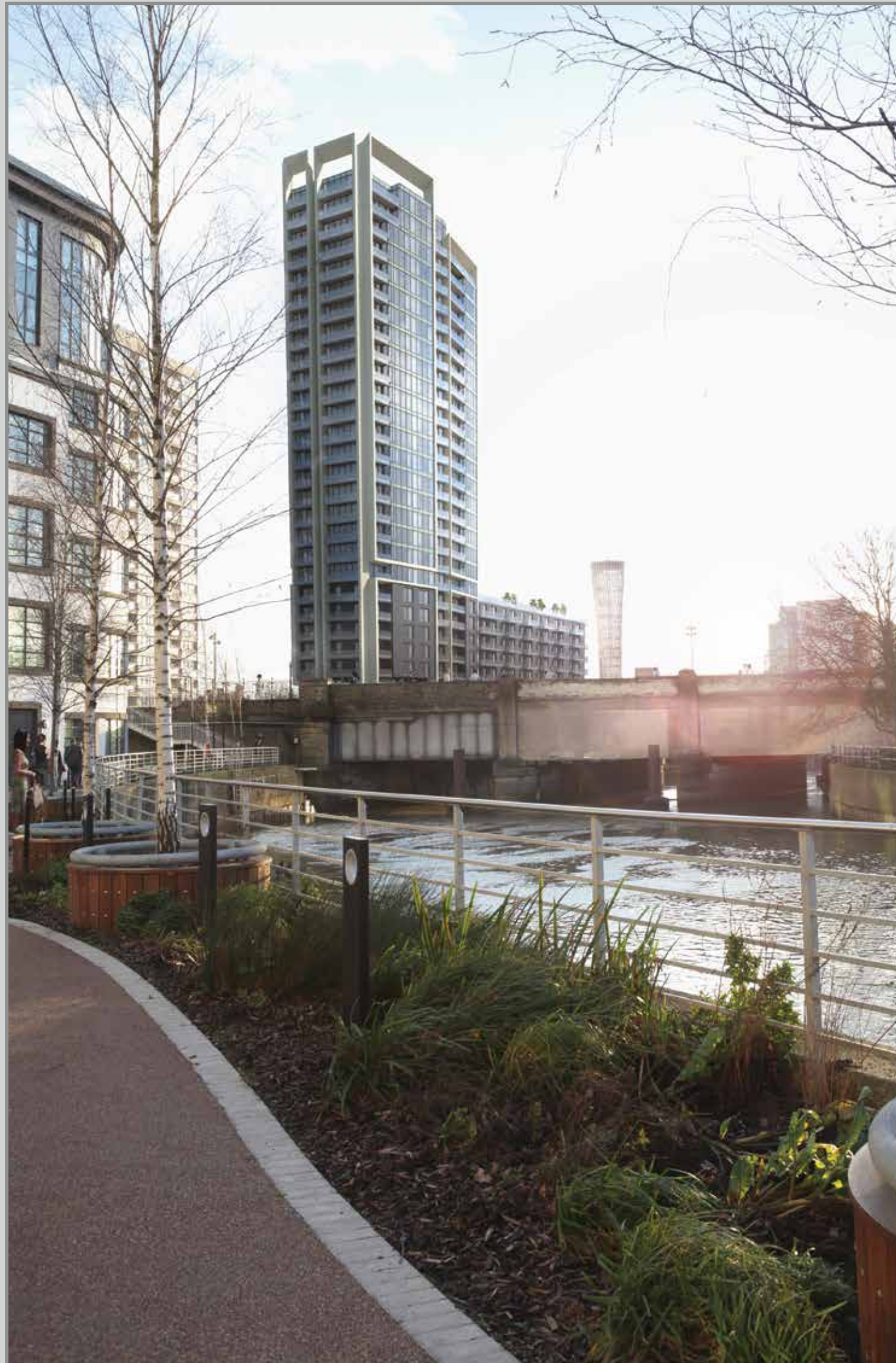
Computer Generated Image of Stratford Riverside exterior, subject to changes during construction process.
