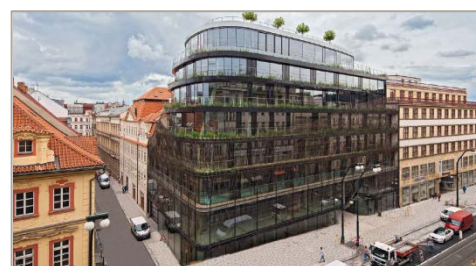
Sebre finished construction of Drn in Prague 1. The building will offer 7 655 sqm of office space.
