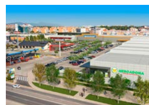
RETAIL PARK TERRASSA PLAÇA Terrassa, Barcelona GLA: 30,535 sqm October 2017
