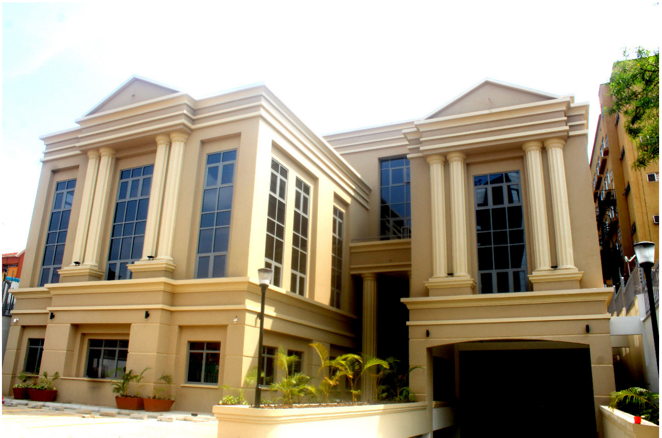
H&G Chambers, Plot 29A, Lumumba Avenue, Nakasero. Office space available to let.
