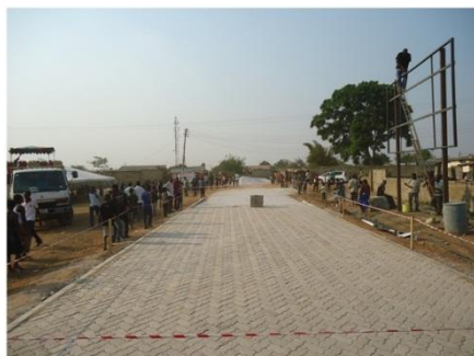
Part of the road constructed using paving stone technology in Chawama Compound
