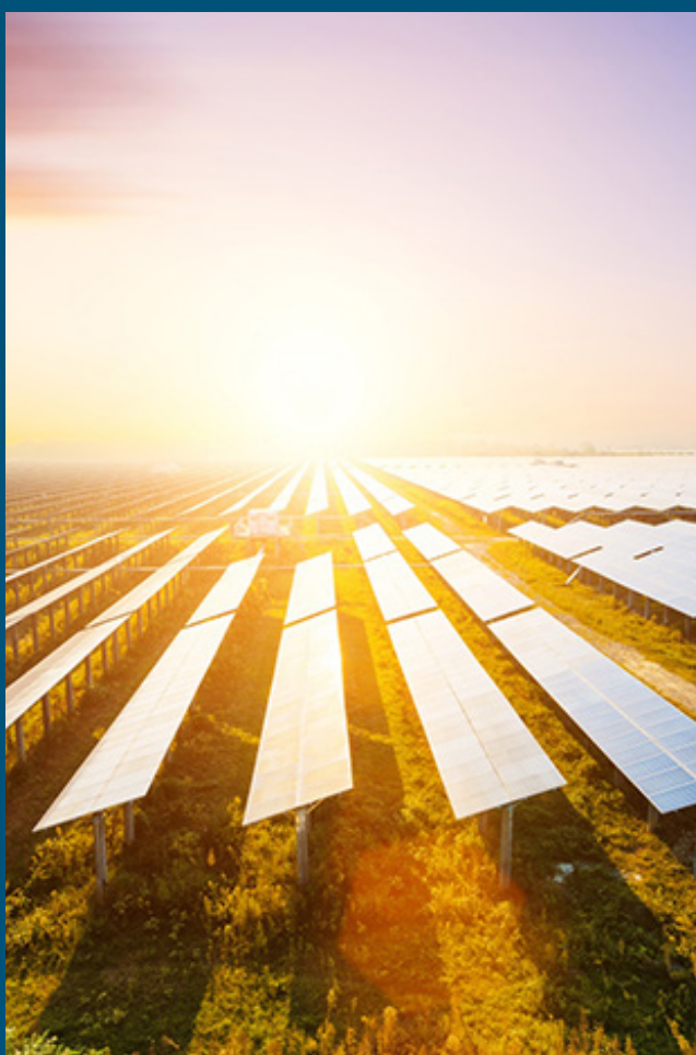
Photo: Bwengu Solar Park Project - Malawi
