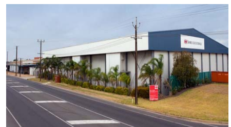
Lot 204 Railway Terrace, Mile End South sold in December 2009 for $4.6 million which represented a building rate of $448/m 2
