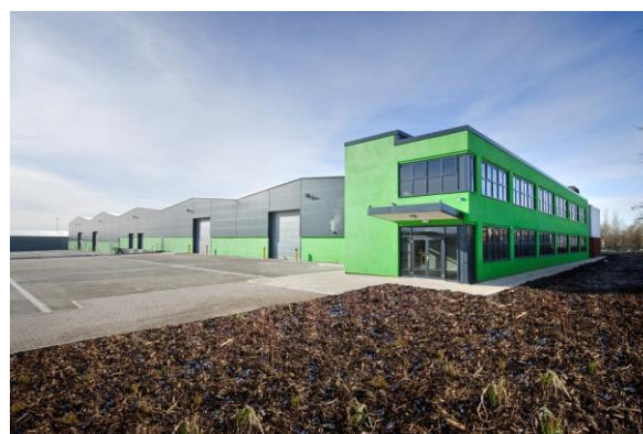
S3 Tyne Tunnel Trading Estate, North Shields (103,950 sq.ft.) recently let to Kitwave Ltd.
