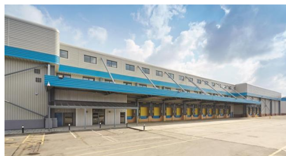
Talke 16, Knight Frank let this 180,000 sq ft refurbished warehouse /distribution/manufacturing at Newcastle-under-Lyme.
