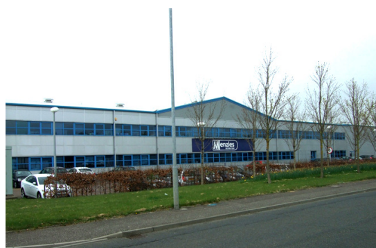
85 Fullarton Drive, Cambuslang Investment Park, Glasgow. Knight Frank acted on behalf of Speedy Asset Services Ltd in their acquisition of this property.
