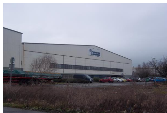
Trident Park, Ocean Way, Cardiff: Knight Frank acted on behalf of Legal & General in selling this 250,000 sq ft warehouse to the Welsh Government. Bad Wolf have subsequently secured a new 10 year lease to use the facility as a studio and office scheme for independent television production.
