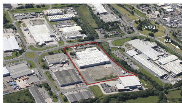
Acting for Bridgend Willis Asset Management Limited Knight Frank acquired this detached Head Quarters facility in Waterton Industrial Estate, Bridgend that measured 123,500 sq ft on a secure site of 9 acres.
