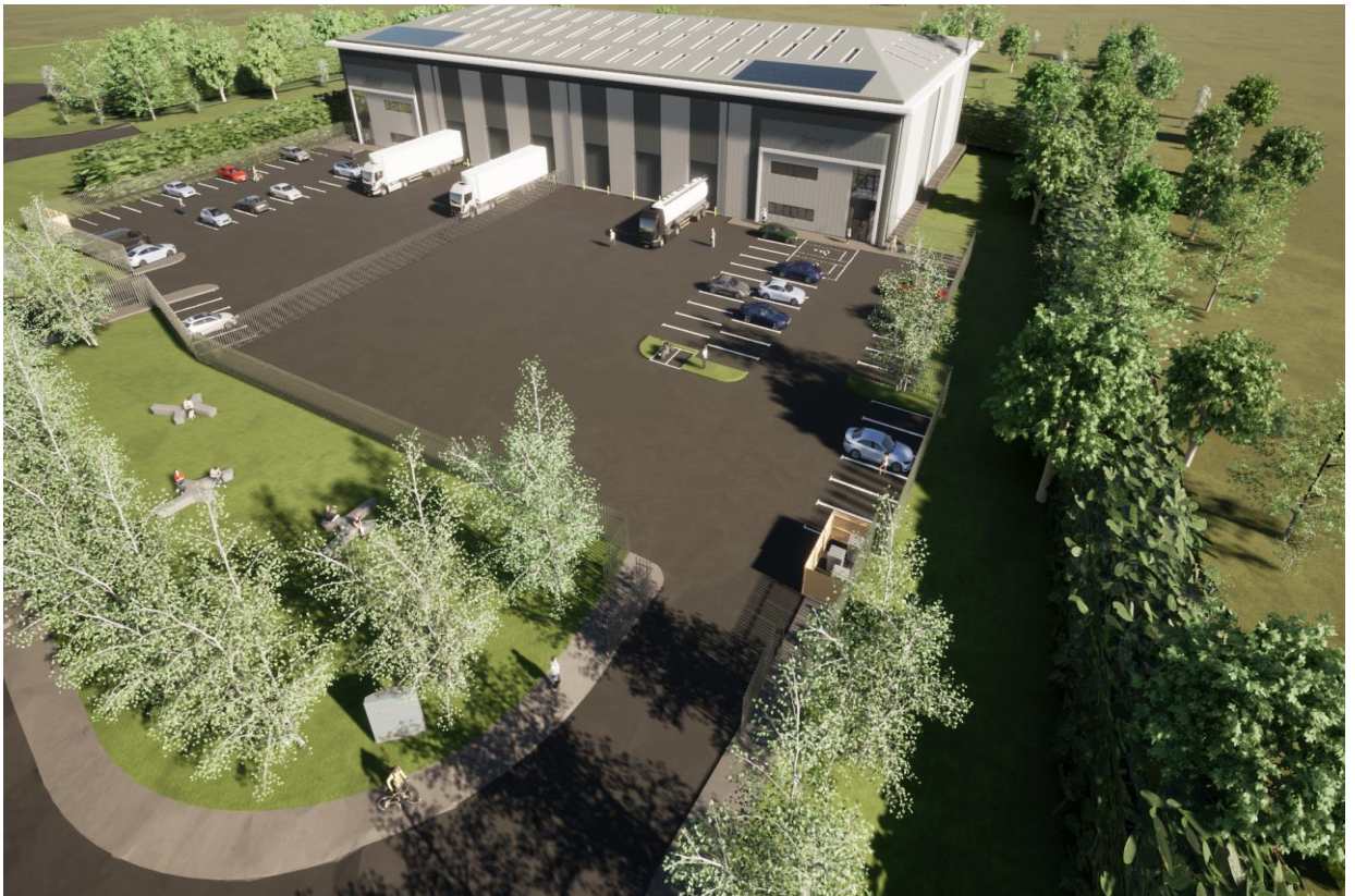
50,000 sq ft new build at Junction 35, Pencoed
