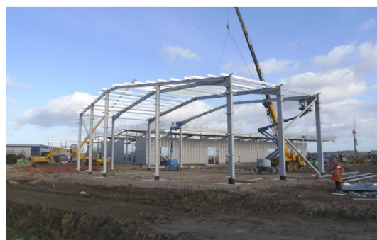
In H2 2011, pallet manufacturer Chep acquired a bespoke 48,525 sq ft unit at Central Park, Bristol. Work is underway with practical completions expected in March 2012.
