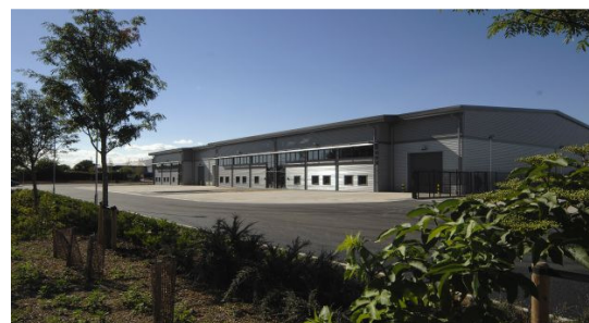
In August 2011, Kelvin Hughes acquired 80,000 sq ft at Canmoor's Voltage building, Enfield, at an agreed headline rent of £8.50 per sq ft.
