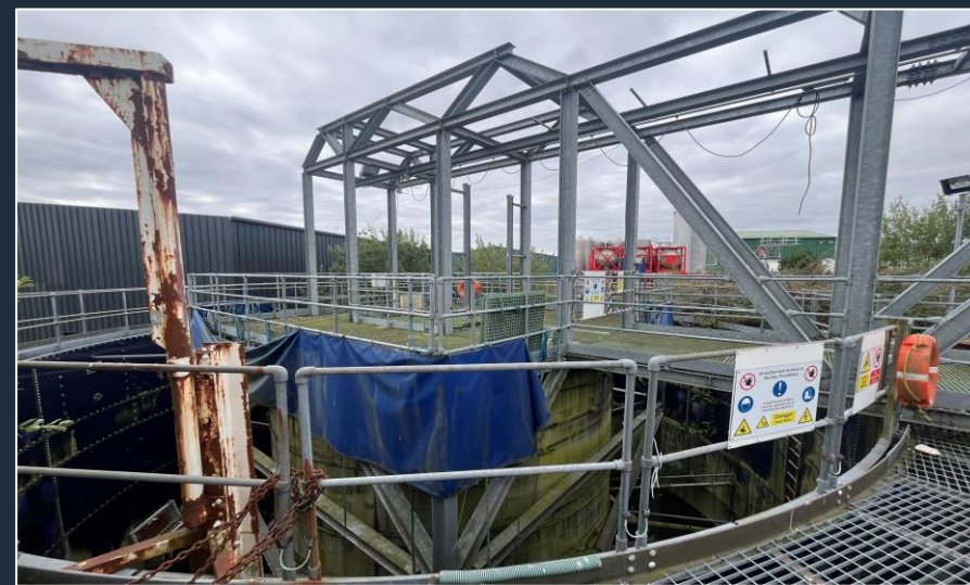
External test pool
