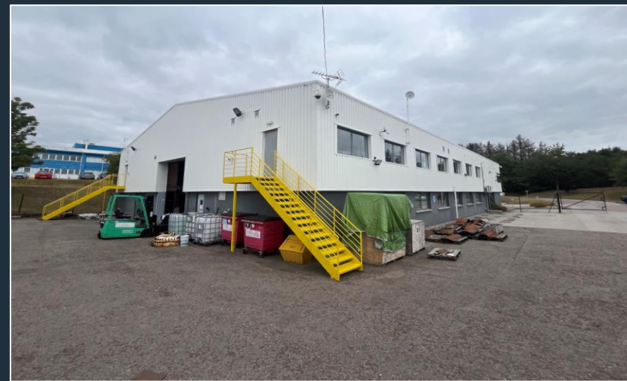
External view from the yard
