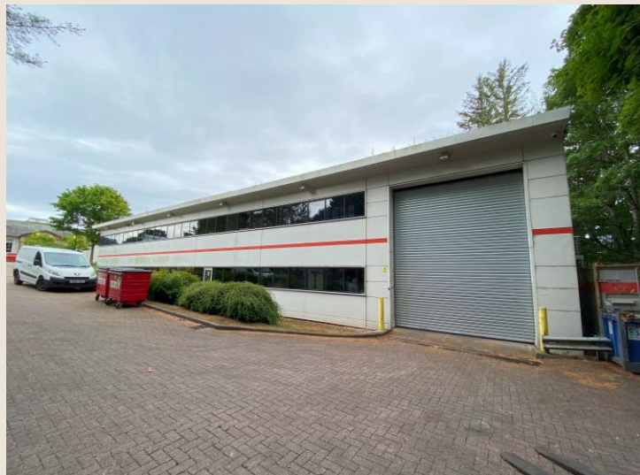
External – Side / Warehouse Access
