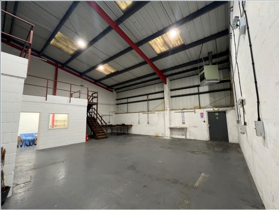
*warehouse currently being refurbished
