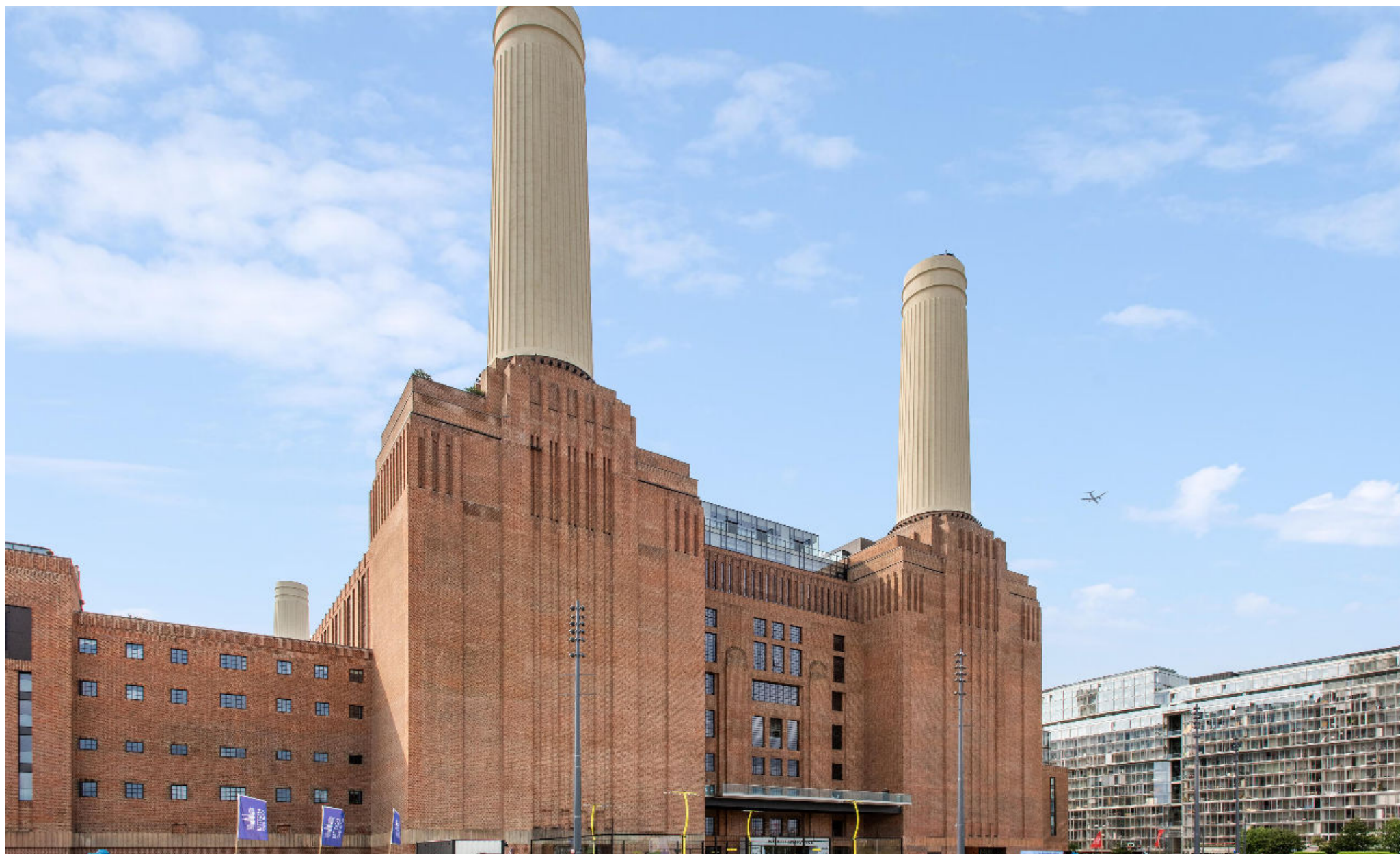
Switch House East, Battersea Power Station SW11
