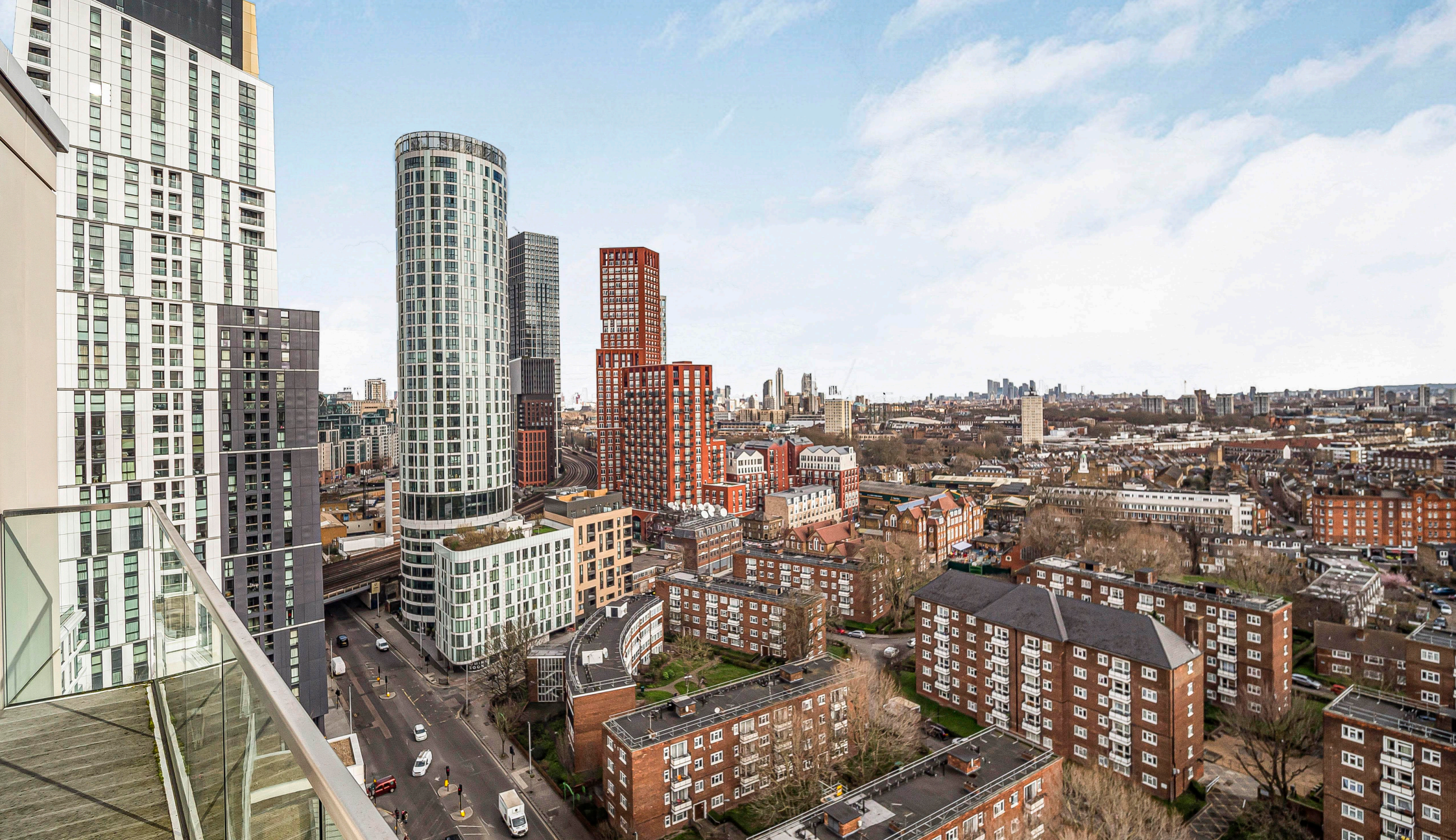
Pinto Tower, Battersea SW8
