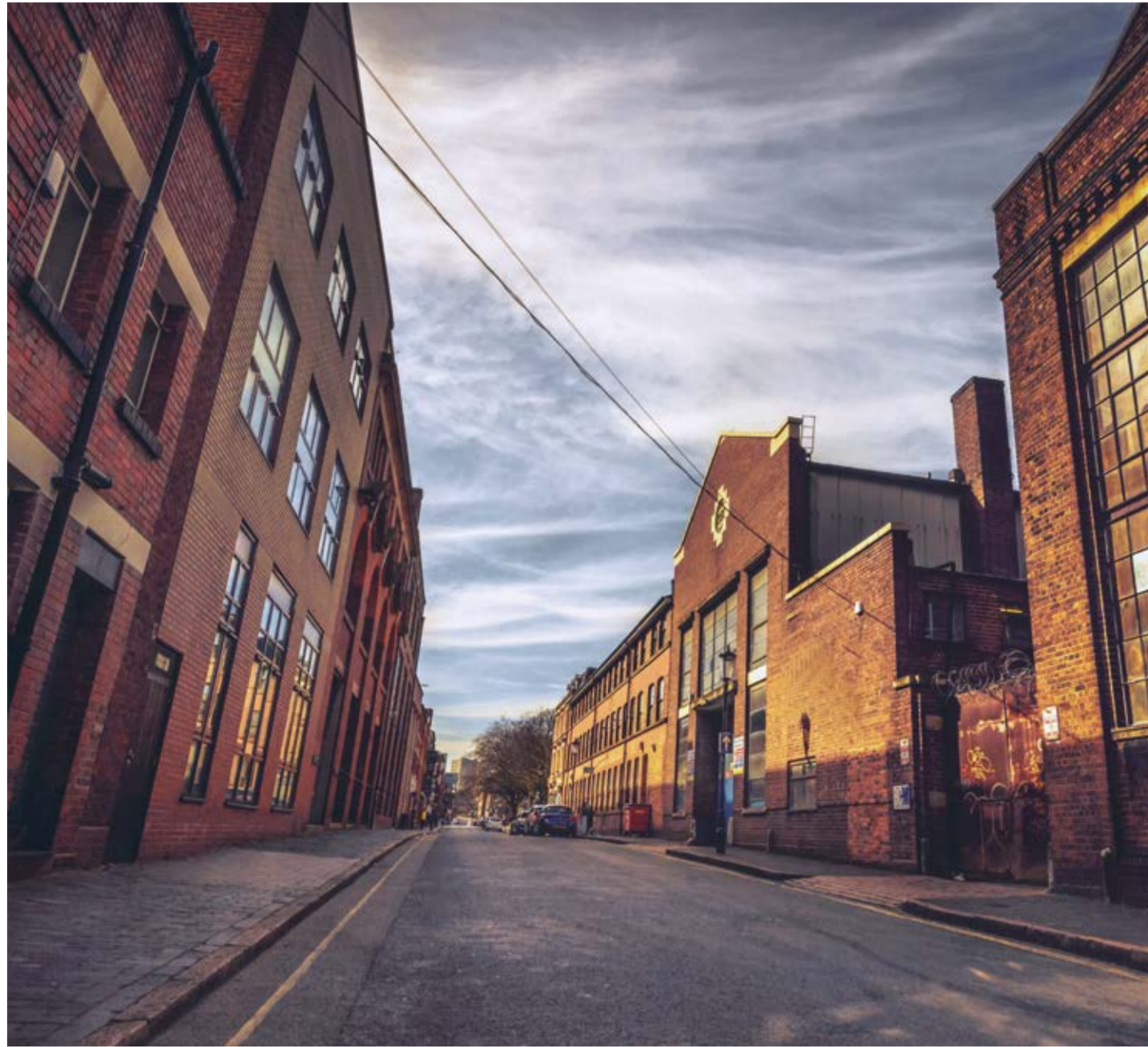
JQ industrial heritage
