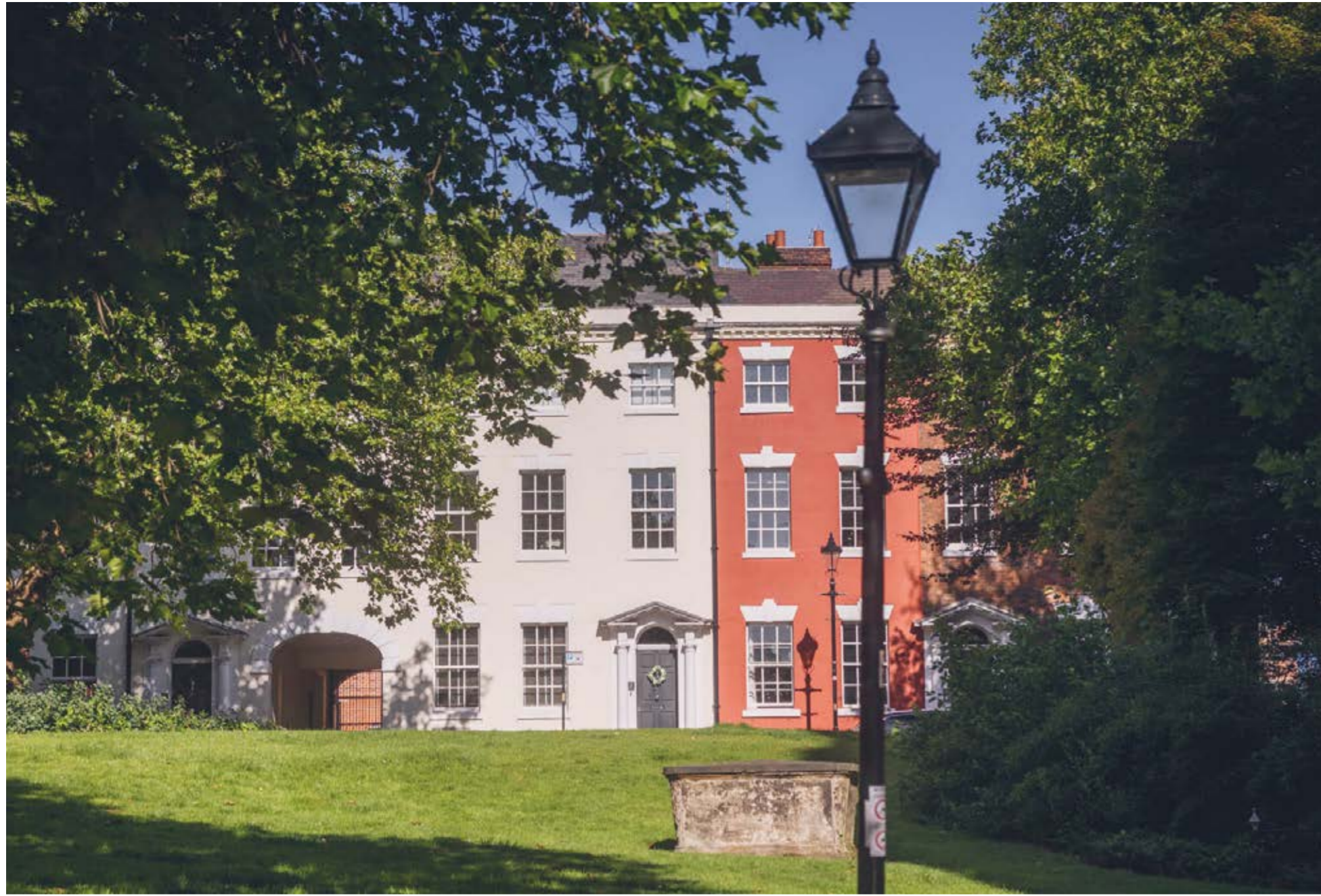
Georgian heritage, St Paul's Square
