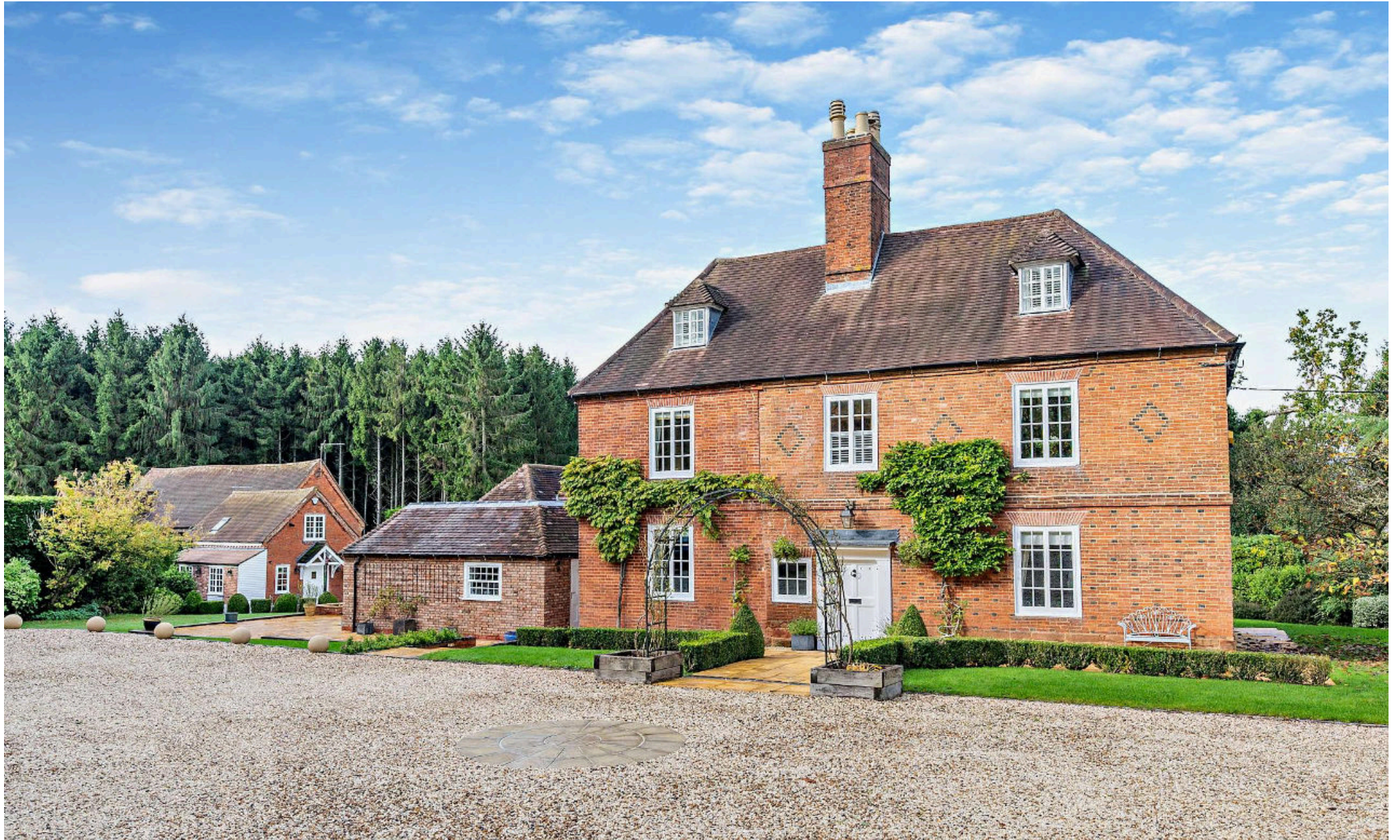
Holly House, Spencers Lane, Berkswell
