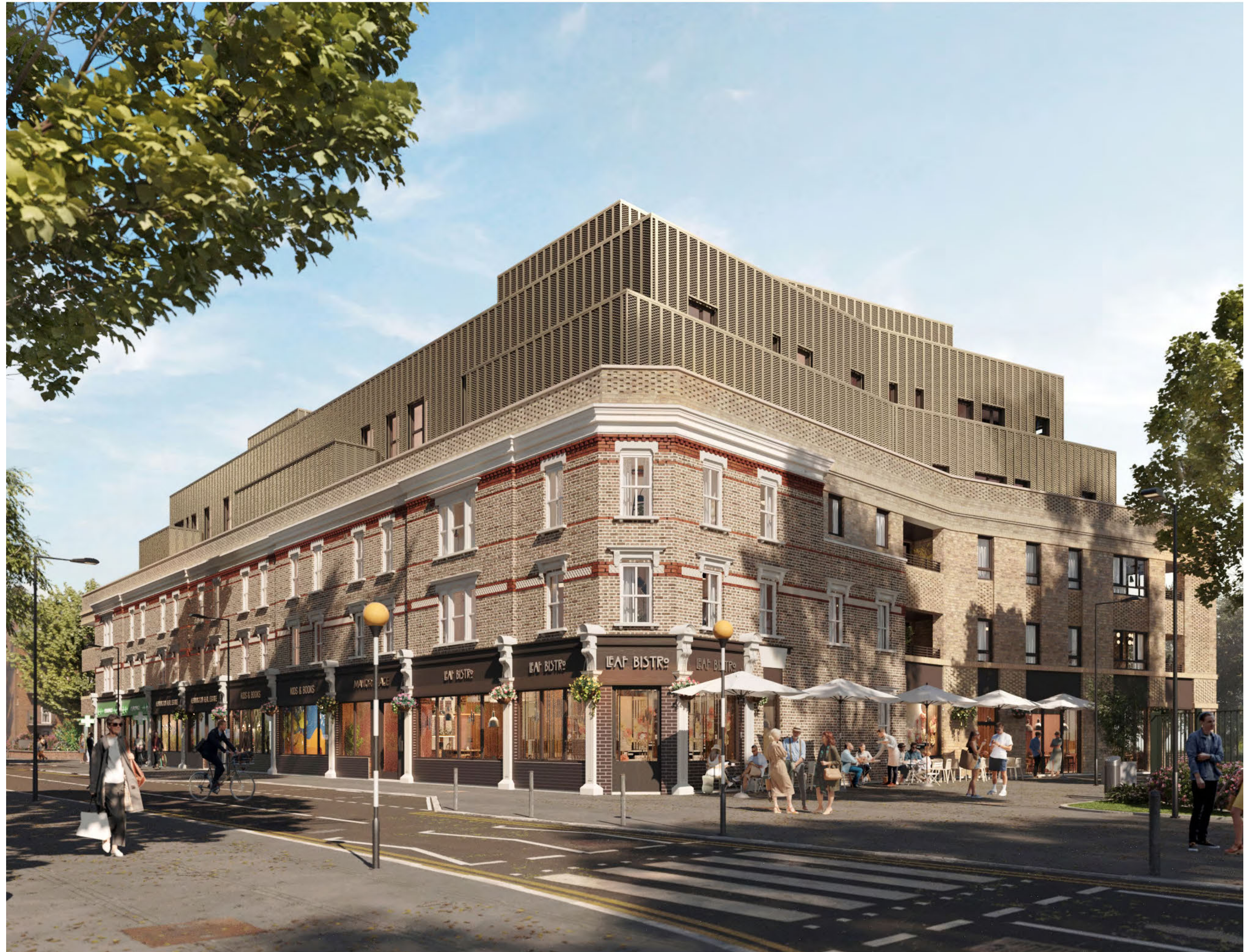
The recreated facade at Manor, with ground floor retail — CGI is indicative only
