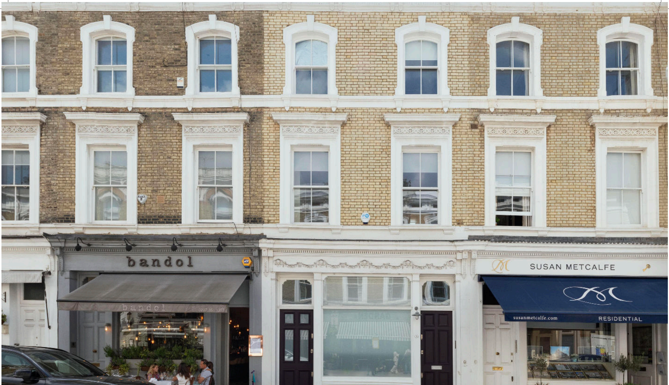
Hollywood Road, London SW10
