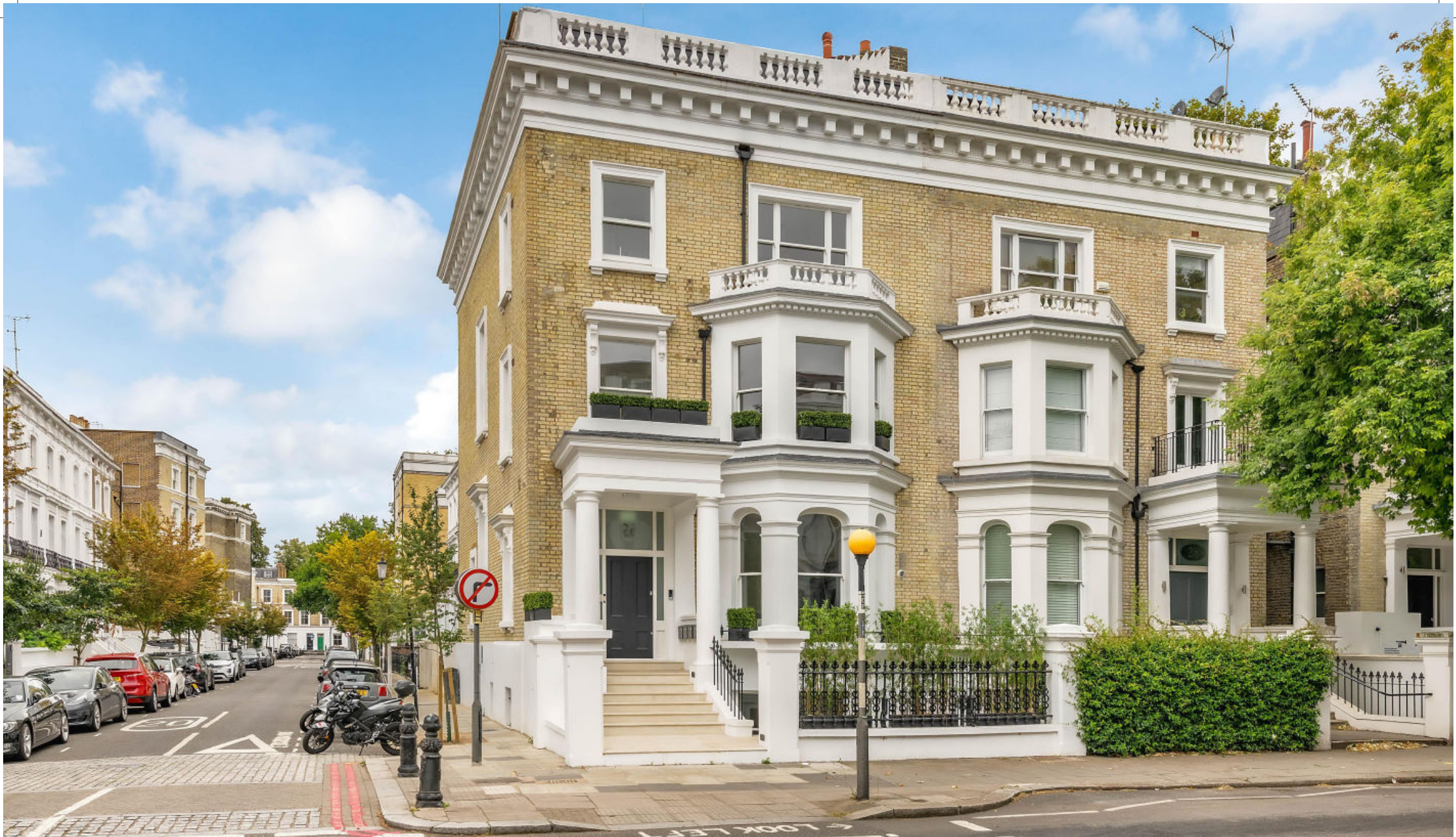
Redcliffe Gardens, London SW10
