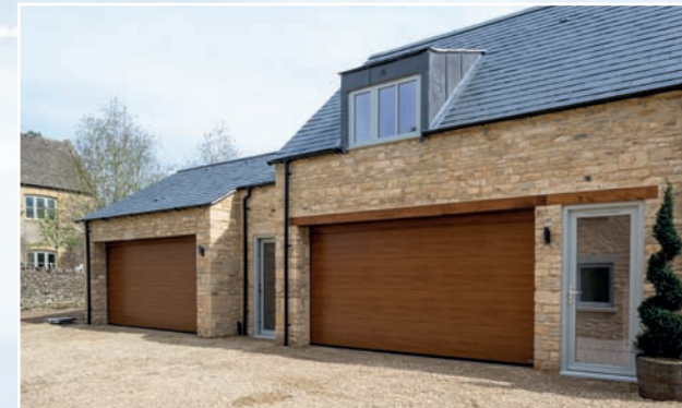
Double garages and entrances to home offices for plots 2 & 3 on opposite side of courtyard.
