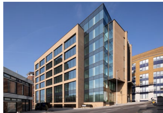
The Brinell Building, Brighton
