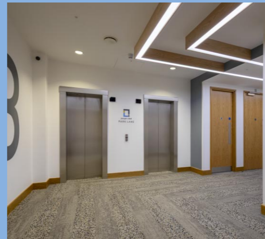
Third Floor Lift Lobby
