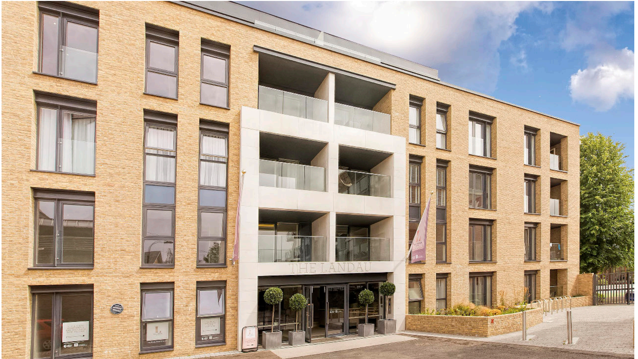
Landau Apartments, London SW6
