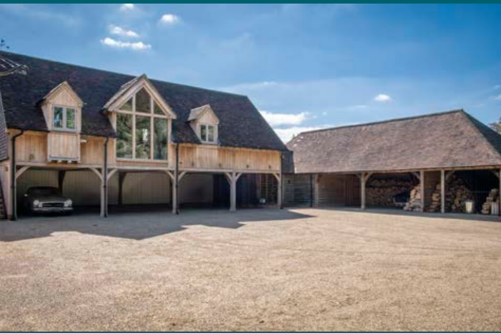
CARPORT AND FIRST FLOOR ROOMS
