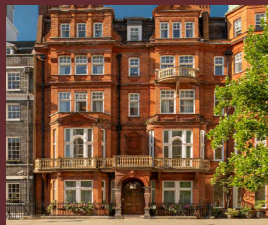
34 BERKELEY SQUARE, W1
