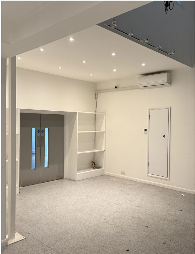
Ground floor warehouse with mezzanine
