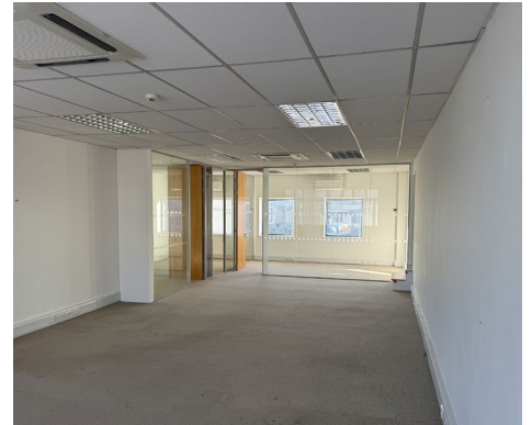
First floor office
