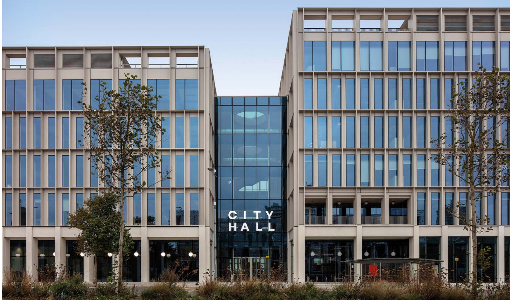
1. The City Hall building
