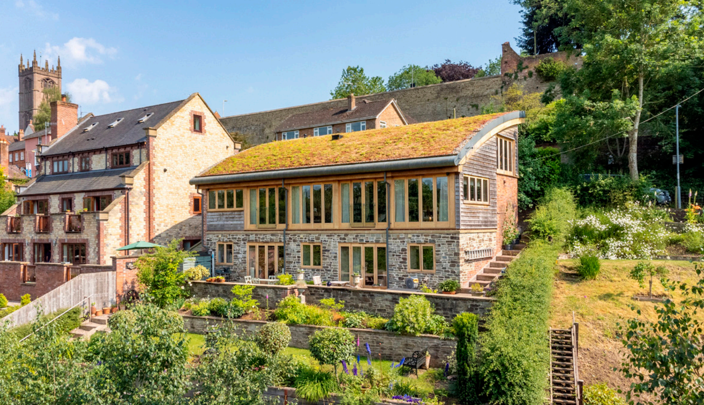
Drawbridge House, Linney, Ludlow, Shropshire
