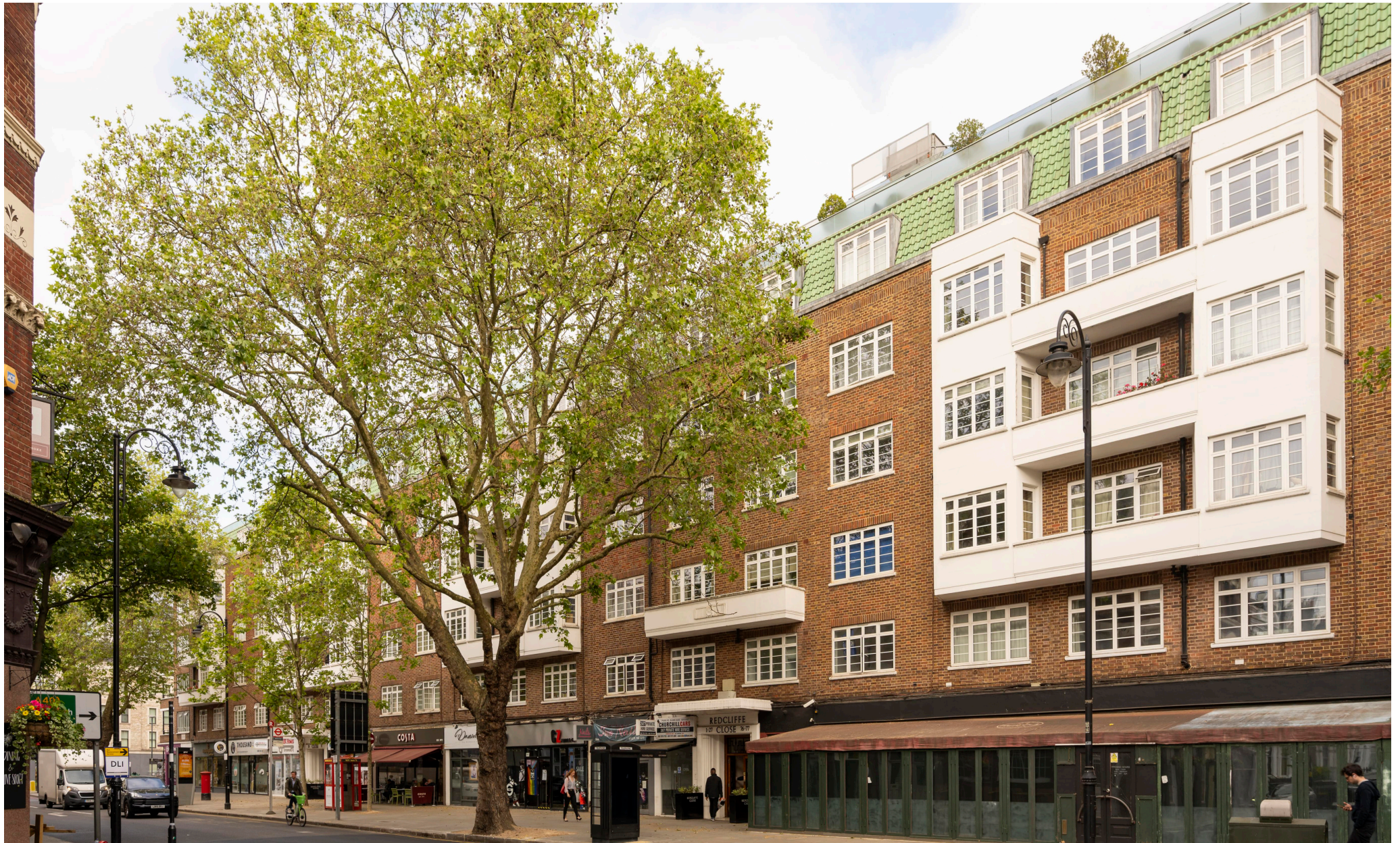
Redcliffe Close, London SW5
