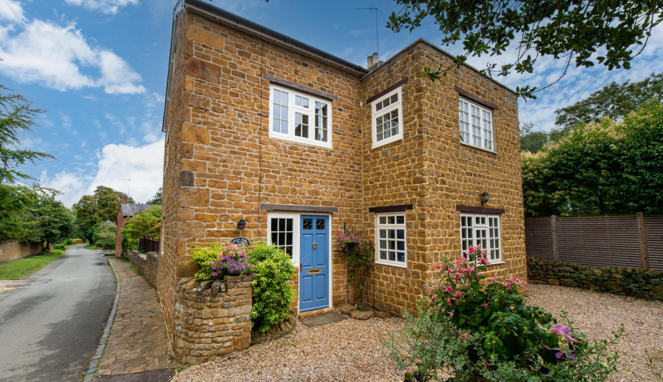
Holly Bush House, School Lane, Warmington
