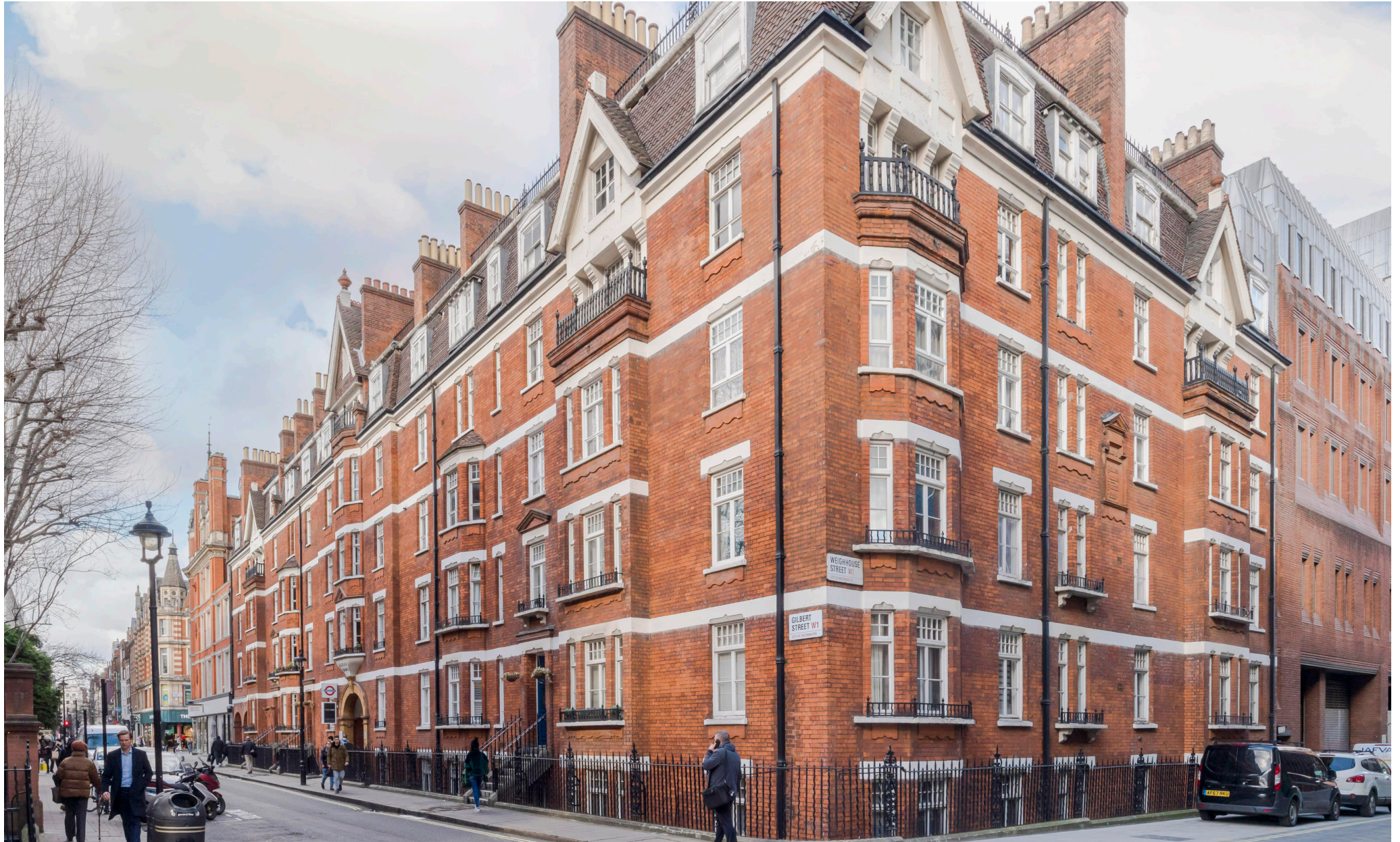
Cavendish Buildings, Gilbert Street W1K
