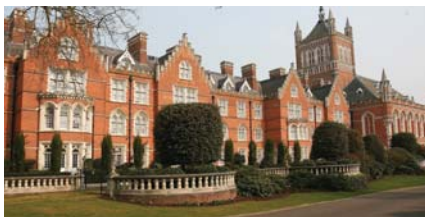
Holloway Drive, Virginia Water
