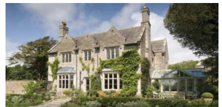
The Old Rectory, Church Knowle
