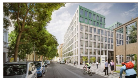
Skanska commenced construction of project Praga Studios in Prague 8. The building will offer approx. 10,600 sqm of office space.
