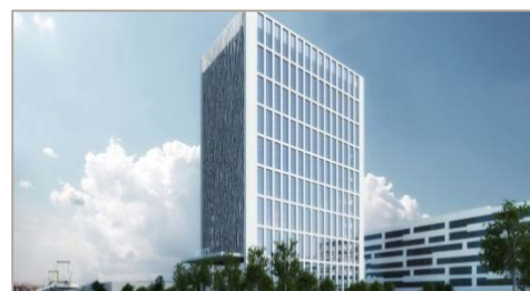
AFI Europe commenced construction of project AFI City in Prague 9. The building will offer approx. 17,000 sqm of office space.
