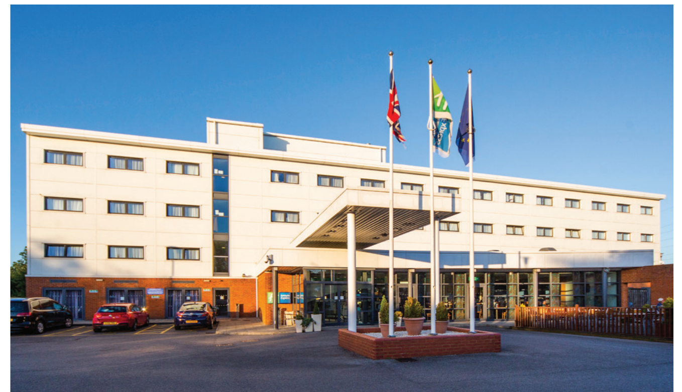
The Holiday Inn Express Folkestone - Channel Tunnel
