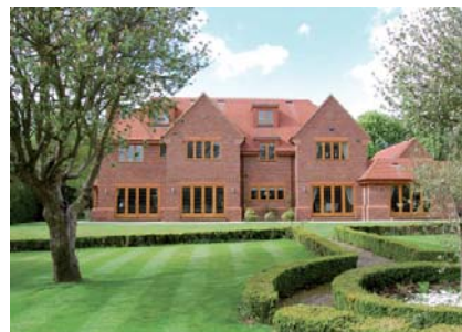
Gerrards Cross, Buckinghamshire New build town house
