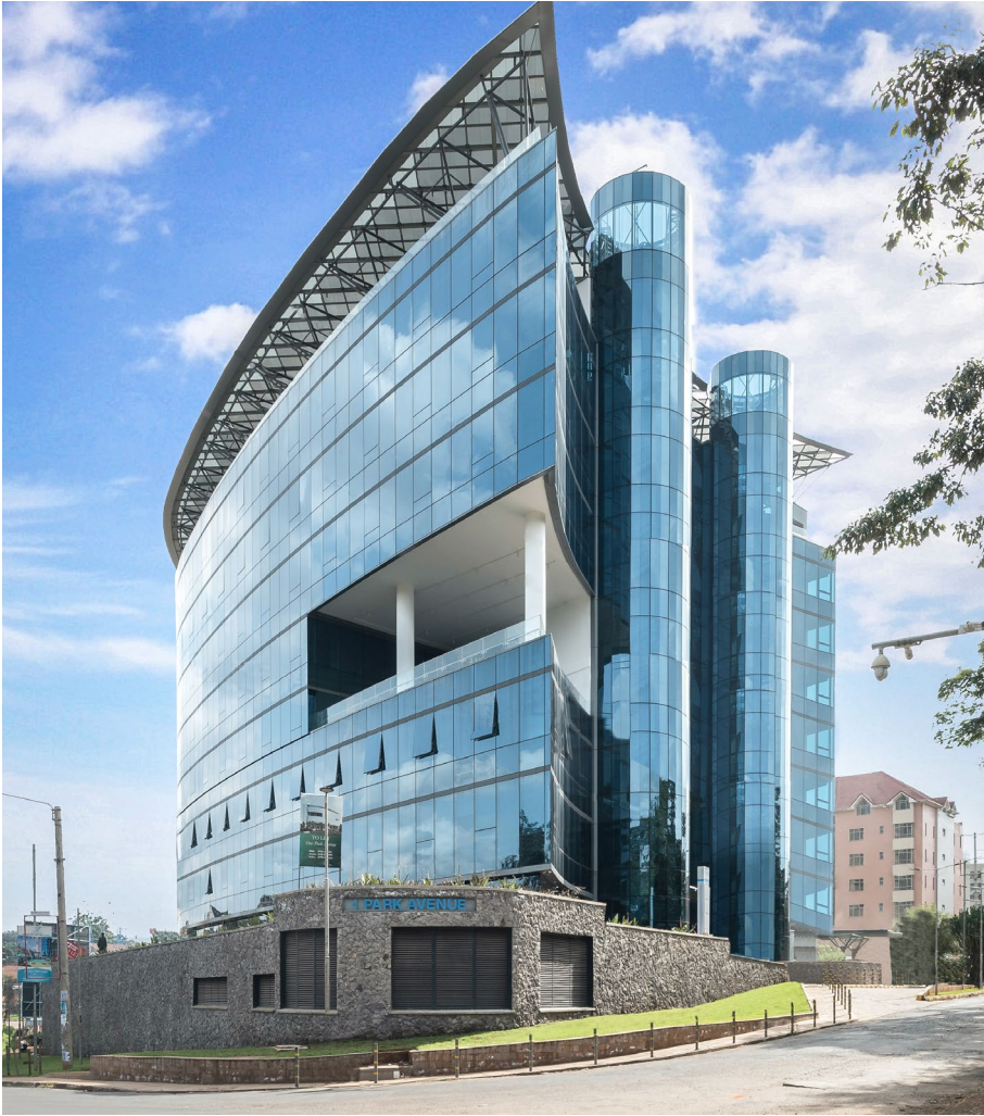
Recently completed 1 Park Avenue in Parklands is currently over 50% let. For more information please contact our Commercial Agency Team.
