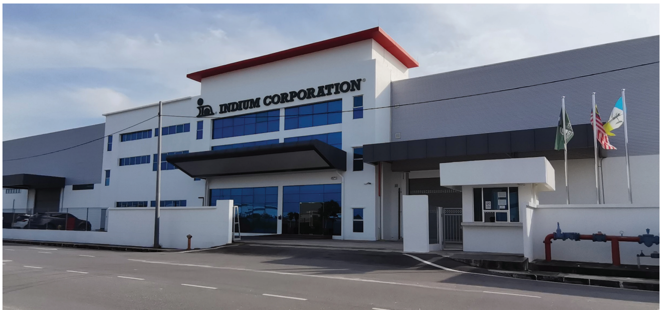
New facility: Indium Corporation in Batu Kawan Industrial Park
