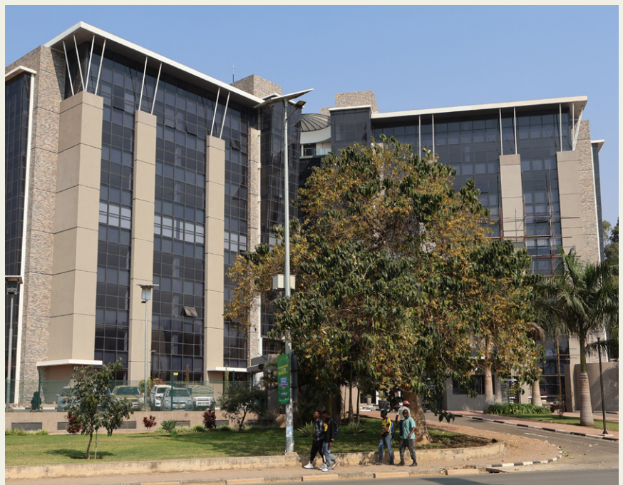
Zepre Office Park, Lusaka, Zambia
