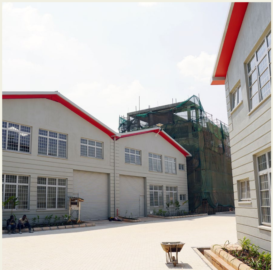
The 65,000 SQM Yogi Business Park in Nalukolongo
