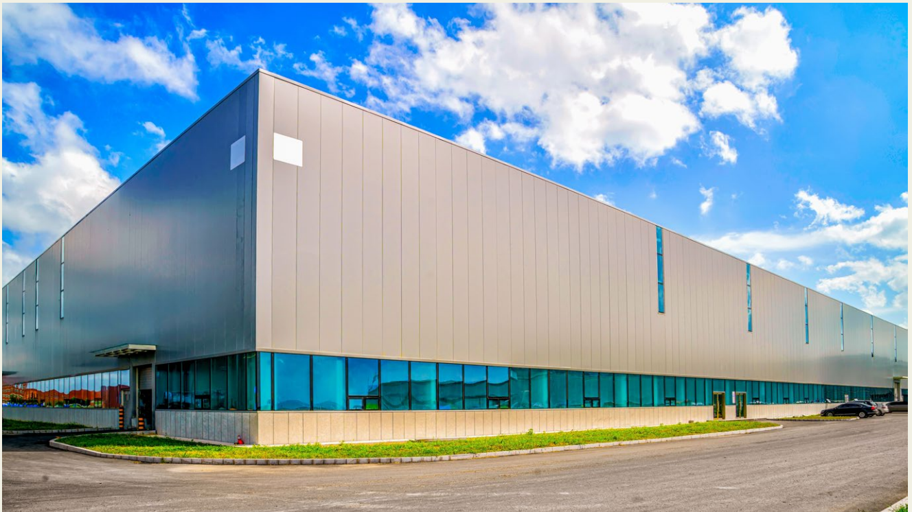
Kahama Industrial Park Shinyanga Region, Tanzania
