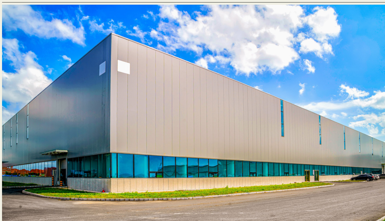
Kahama Industrial Park Shinyanga Region, Tanzania
