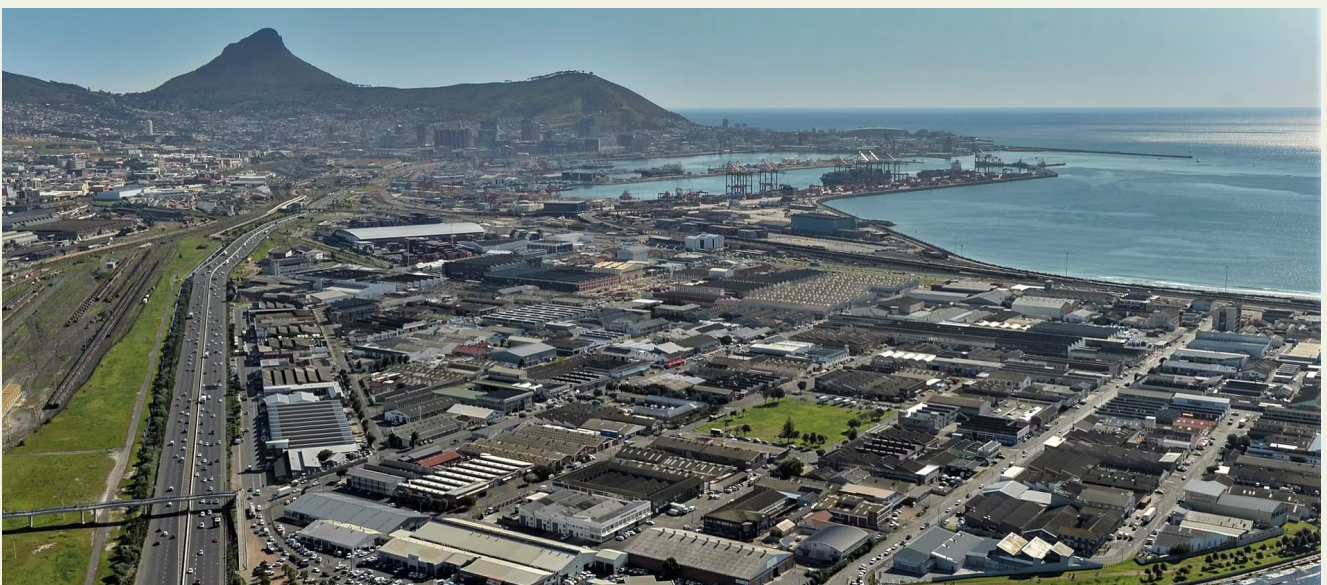
Cape Town Industrial Zone
