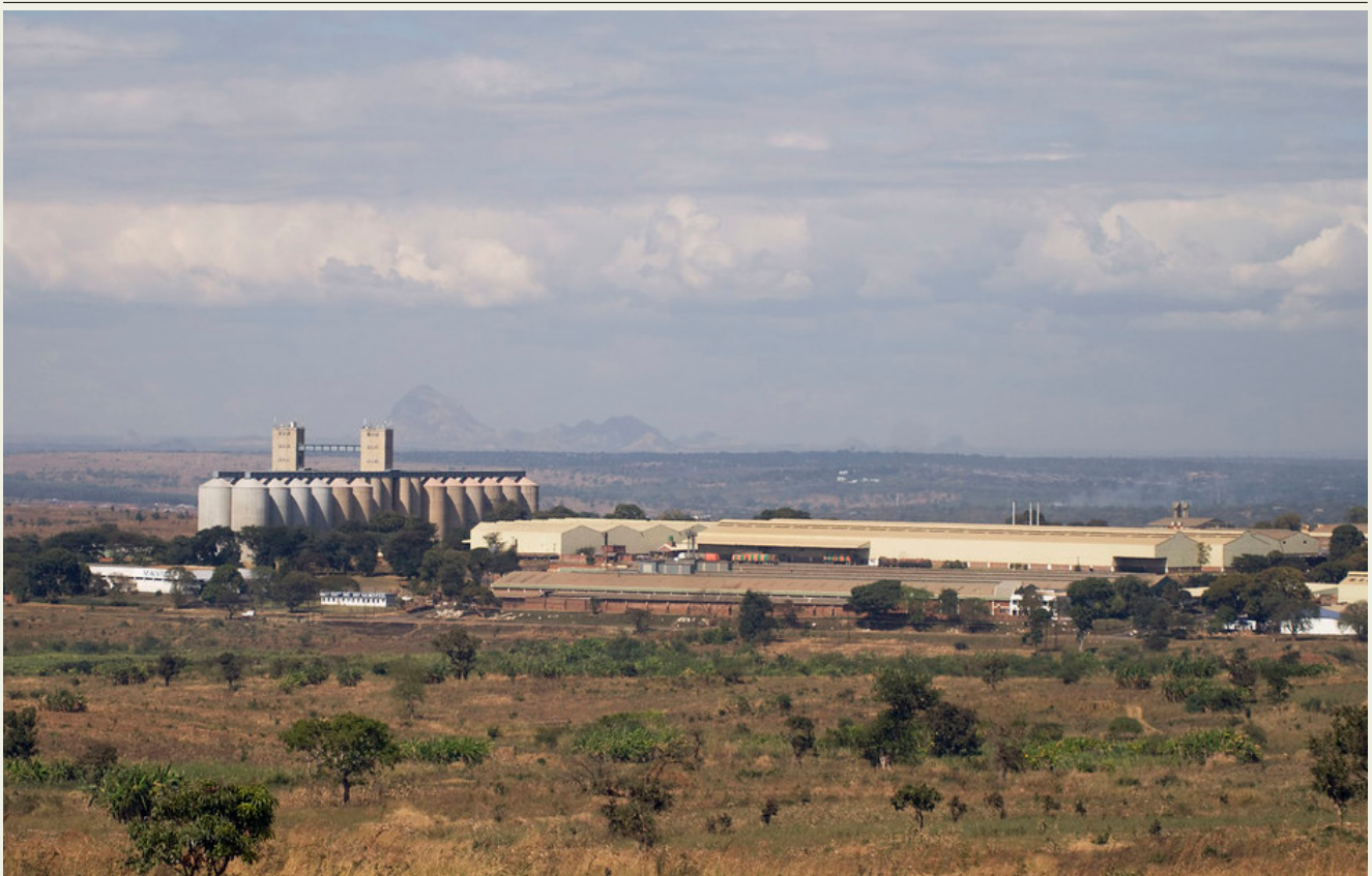
View of the Kanengo Silos Complex, a large grain storage facility located on the outskirts of Lilongwe, Malawi
