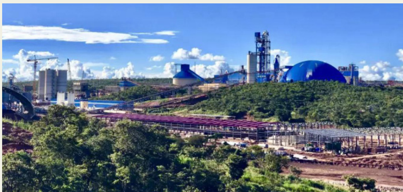
A view of CNBM-Zambia Industrial Park (COURTESY OF CNBM)
