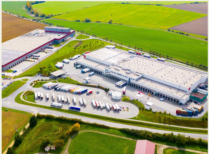
Kahama Industrial Park Shinyanga Region, Tanzania
