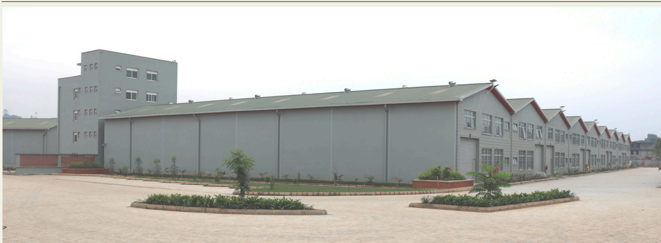
The 65,000 SQM Yogi Business Park in Nalukolongo
