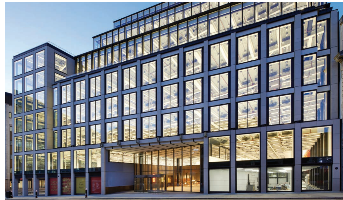
The JJ Mack Building, Farringdon
