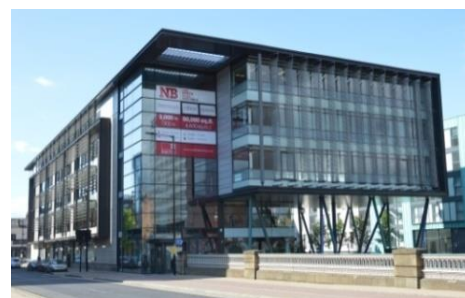
XLC Telecom moved into Northbank in October 2014 and secured an additional 14,000 sq ft of city centre office space in July 2015
